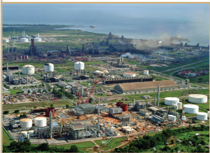
Methanol plant at Point Lisas
