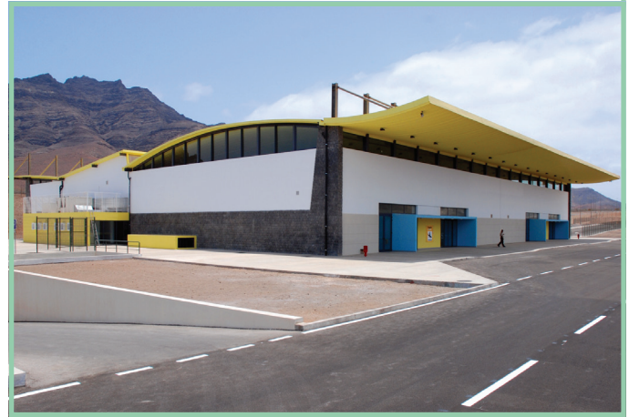
The final step for the certification of São Vicente's airport for international flights is underway.
