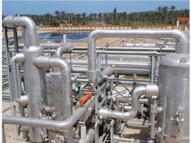
Dana Gas Egypt's El Wastani gas-processing facilities in the Nile Delta. www.danagas.com
