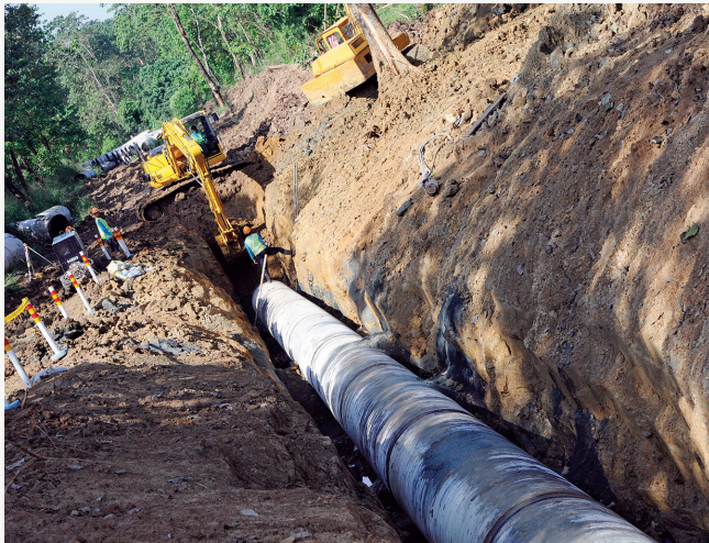
Pipeline project by M.E. Sicat Construction
